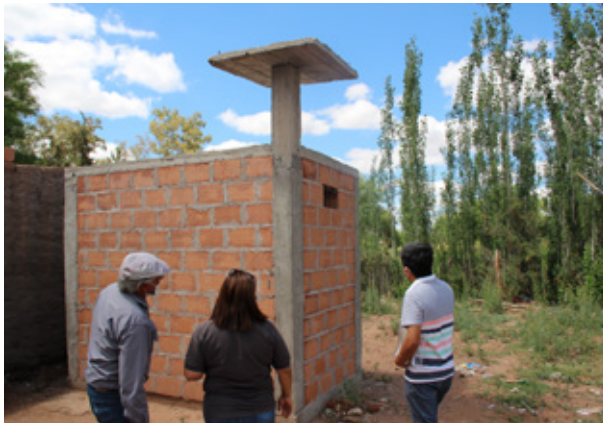
Elimination of latrines. Jáchal, Argentina
