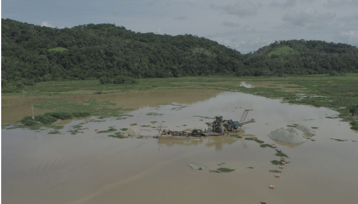
Figure 16-11: Floating Excavator/Plant Mining Cargueros Dredge Tailings
