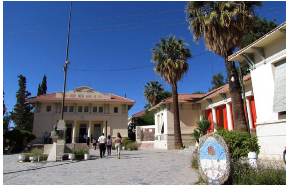
|||| Maintenance of Fray Justo Santa María de Oro School, which is 104 years old
