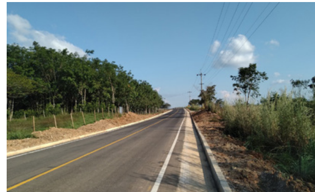
||| Escorralao Road, after being paved
