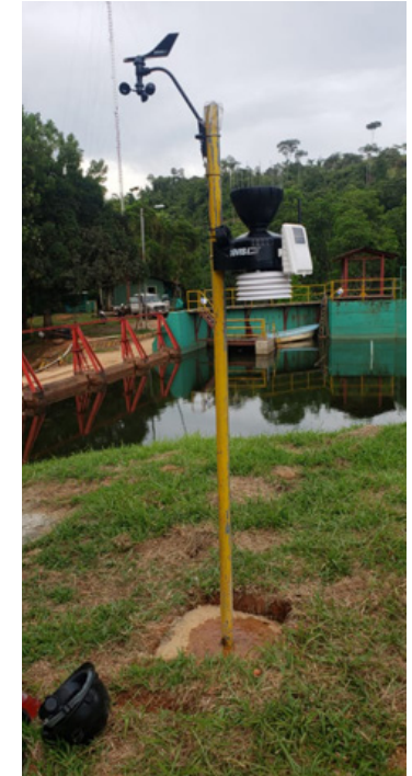
Meteorological station at the Siempre Viva Hydroelectric Plant
